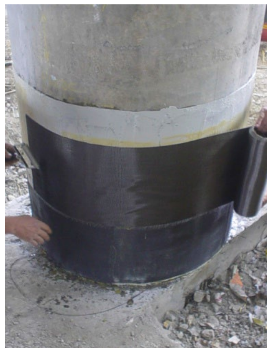
Figure 4. Confinement strengthening [5]
