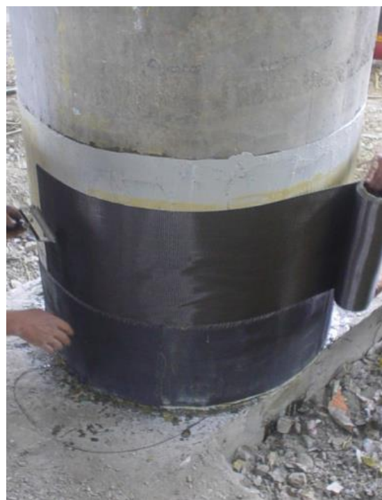
Figure 4. Confinement strengthening [5]
