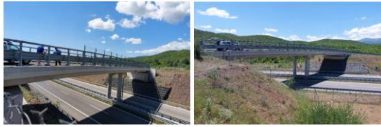
Figure 2. Measured structures OP2 and OP3
