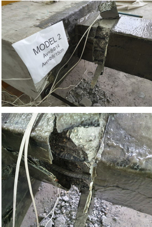
Figure 10. Observed damages during the quasi-static testing of Model M2.
