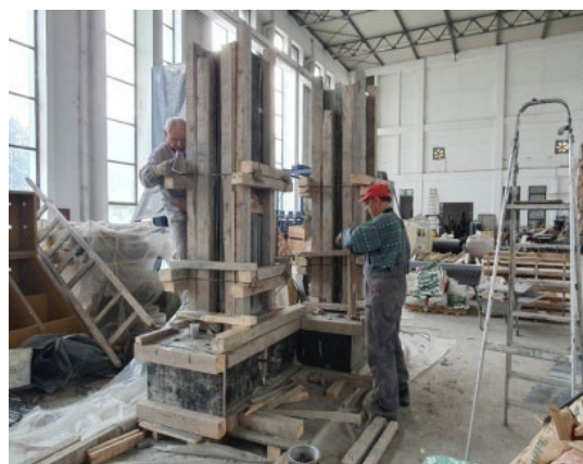
Figure 2a. Construction of the column models for experimental tests
