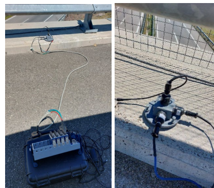
Figure 1. Field monitoring equipment (left), three-way accelerometer (right)
