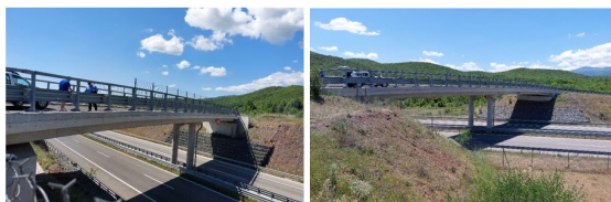
Figure 2. Measured structures OP2 and OP3
