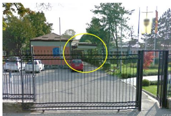
Figure 9. Photograph of the canopy on the building shown in Figure 8
