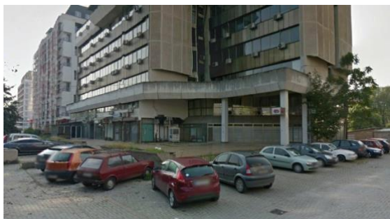
Figure 15. Photograph of the building shown in Figure 13 – north side
