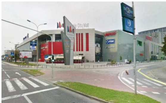
Figure 11. Photograph of the building shown in Figure 10 - Skopje City Mall
