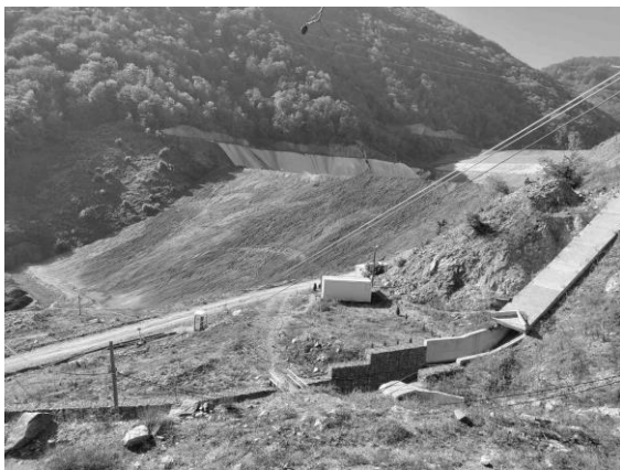
Figure 4. Downstream slope of tailings dam Sasa 4. Picture dates from October, 2022
