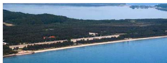
Figure 1. View Prora complex [1]
