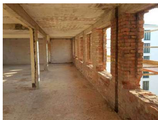
Figure 8. Interior under reconstruction
