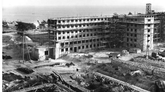
Figure 6. Building under construction [2]
