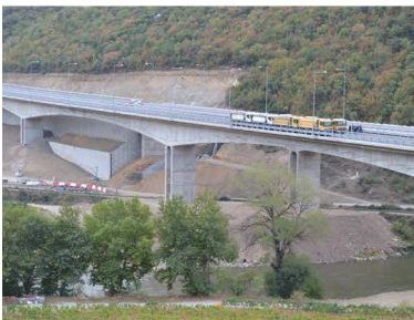
Static and dynamic proof loading tests on roadway concrete bridges
