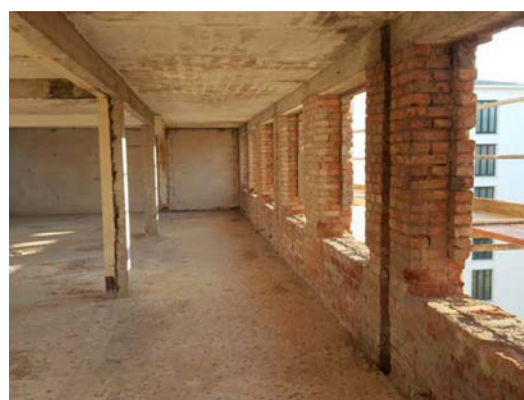
Figure 8. Interior under reconstruction
