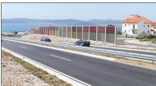
Figure 3. Absorbing concrete barrier at the entry to the City of Zadar (2007), [10]
