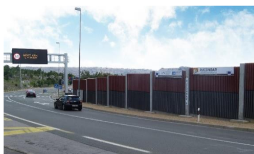
Figure 11. First application of RUCONBAR noise barriers on road section (noise road protection of the settlement Scott)
