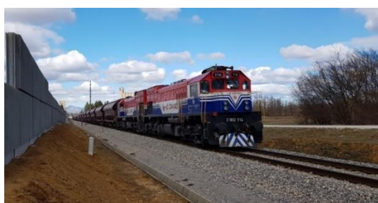
Figure 12. First application of RUCONBAR noise barriers on railways line (noise protection of the settlement near railways station Gospić)
