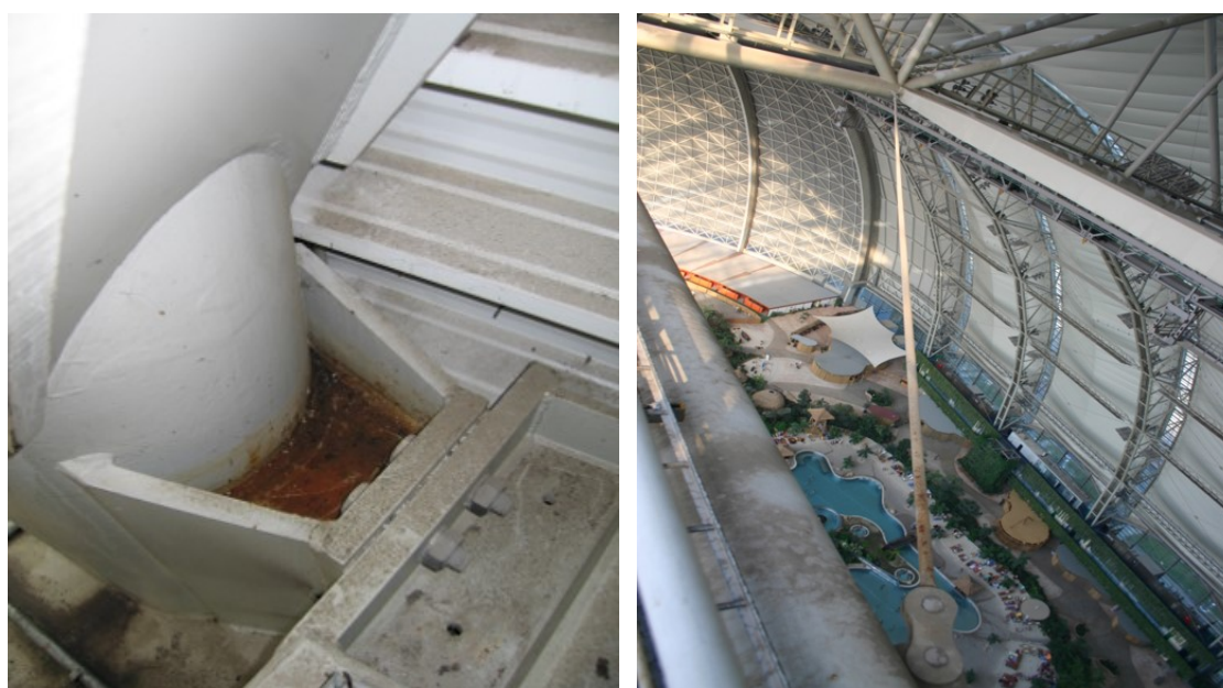
Figure 3. Some inspection results
