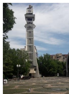
Figure 2. View of the bell tower
