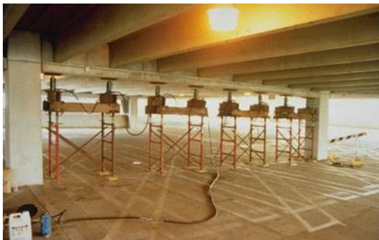
Figure 5. Hydraulic test loading
