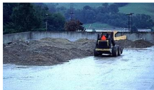
Figure 20. Excessive construction loads
