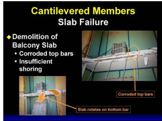
Figure 23. Balcony slab failure
