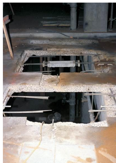
Figure 15. Compression struts in post-tensioning repairs
