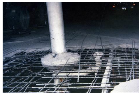
Figure 19. Removing concrete around column
