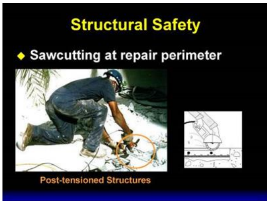
Figure 22. Cutting post-tensioning tendons
