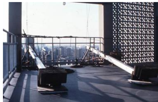
Figure 4. Supports for suspended scaffold
