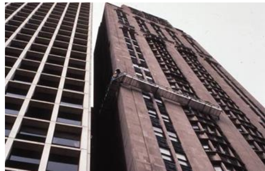
Figure 3. Suspended scaffolds on the side of the building
