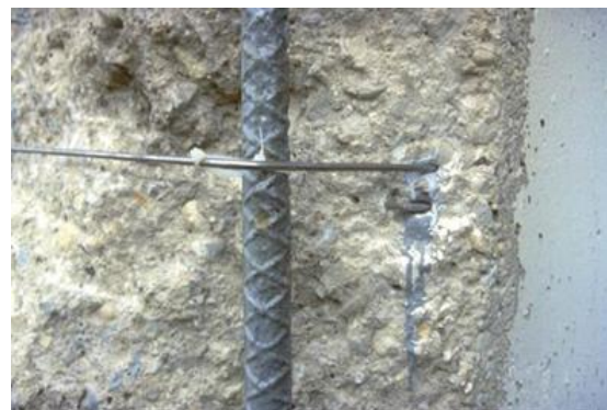
Figure 21. Facade patch repair
