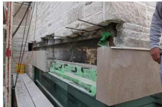
Figure 13. Repair of steel shelf angle/window lintel
