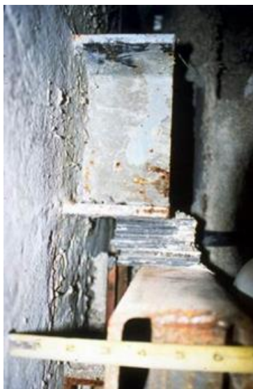
Figure 14. Failure of facade panel connection
