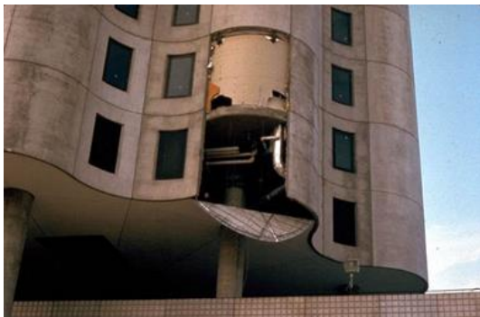
Figure 14. Failure of facade panel connection
