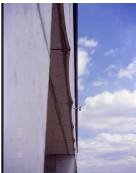
Figure 26. Bowing of panels
