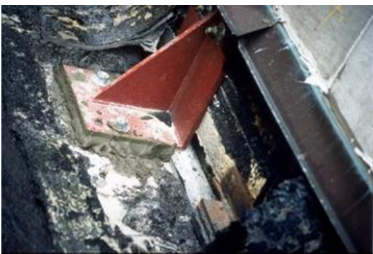
Figure 18. Connection retrofit with steel bracket
