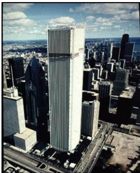
Figure 25. Recladding of the 82-story tall marble clad Amoco building
