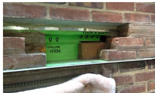
Figure 7. Repaired steel lintel with installed flashing over it
