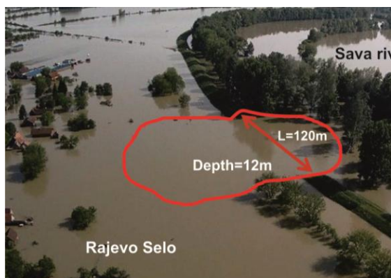
Figure 5. Breach of a Sava River dyke with an extensive scour on the landside (120 x 300 x 12m) due to internal erosion of the ground below the dyke. (Croatian Ministry of Agriculture, 2014)
