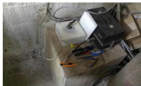
Figure 3. Installation of the seismic monitoring network
