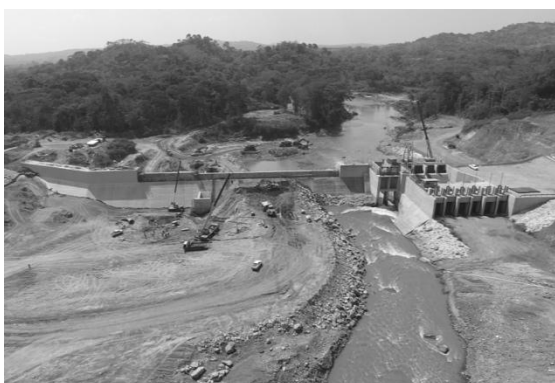
Figure 8. Deep grouted anchors used at the Panama Canal Water Saving Basins and at Ambarau dam
