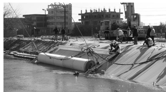
Figure 9. SIBELONMAT® installed underwater at Ismailia canal, Egypt 2016
