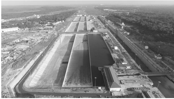
Figure 7. Murdhari GFRD (left) and 9 of the 18 Water Saving Basins of the Panama Canal Expansion
