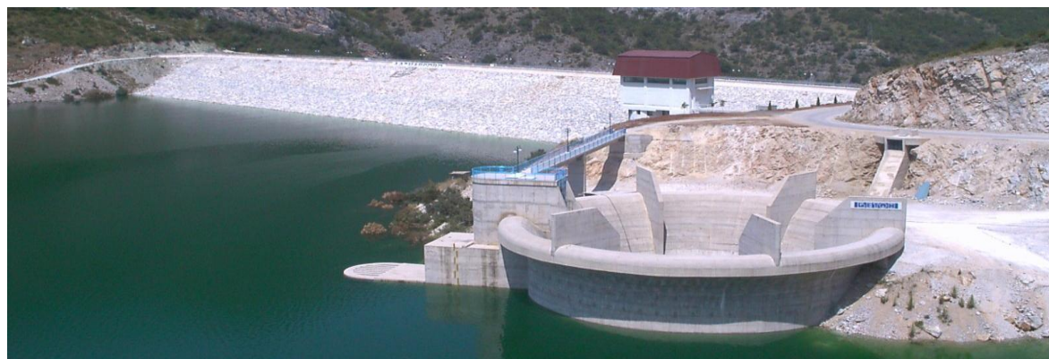
Figure 8. Upstream view of Kozjak dam, highest earth-rock dam in R Macedonia
