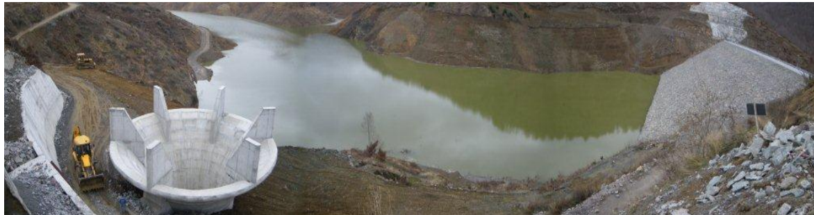
Figure 7. Rockfill dam Knezhevo with asphalt core, on river Zletovska, built in 2011 with structural height of 82 m
