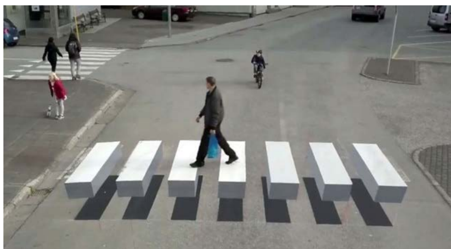
Figure 14. 3D pedestrian crossing as a means to increase pedestrian safety on roads [10]
