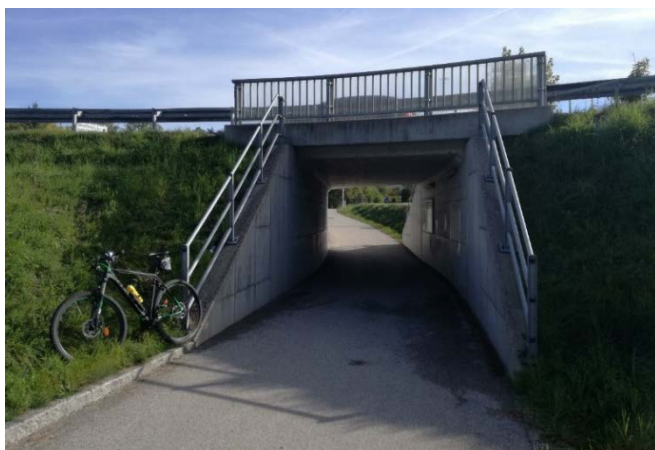
Figure 8. Underpass for cyclists KV „Lenzing South“ [author]
