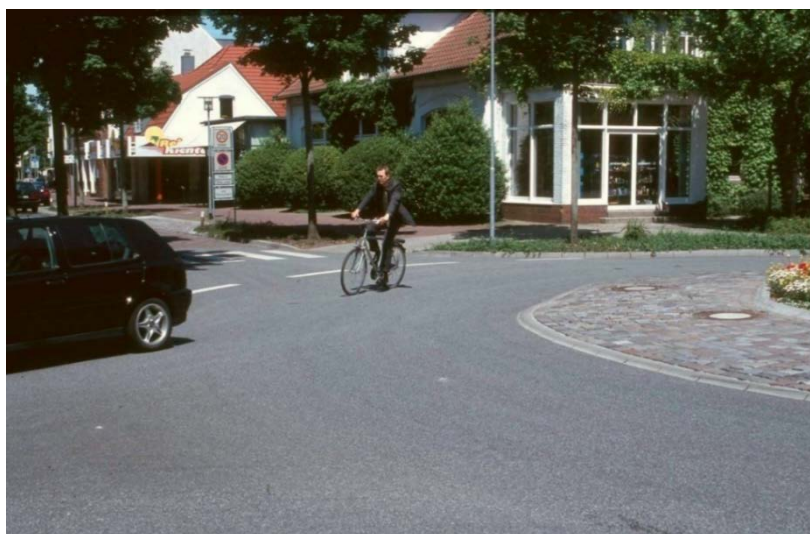
Figure 2. Bicycle routing in the area of a small roundabout on the circular carriageway - recommendation up to 15,000 vehicles / 24 h [1]
