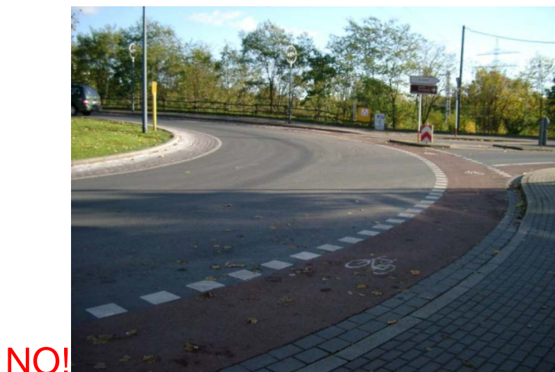
Figure 3. Directions of bicycle traffic on a special bicycle path on the roundabout - the safety of cyclists is significantly endangered! [1]
