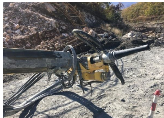
Figure 2. Robot machine for embedding sprayed concrete
