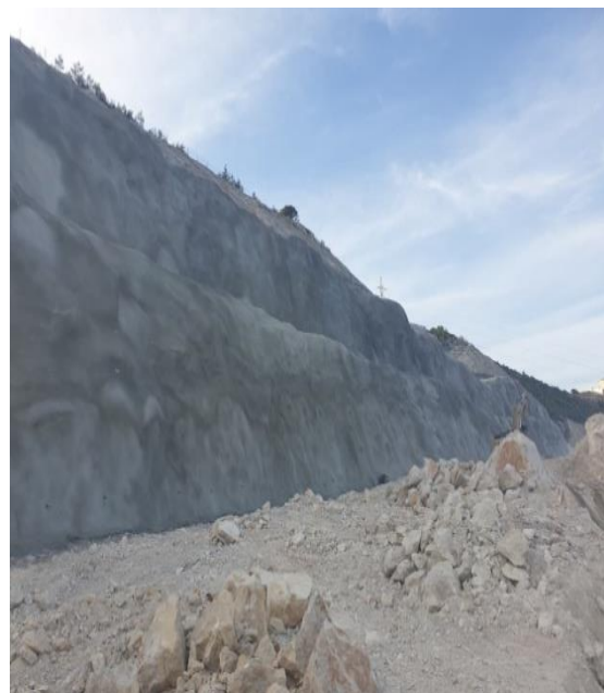
Figure 4. Protection of slopes, on the expressway Prilep - Gradsko
