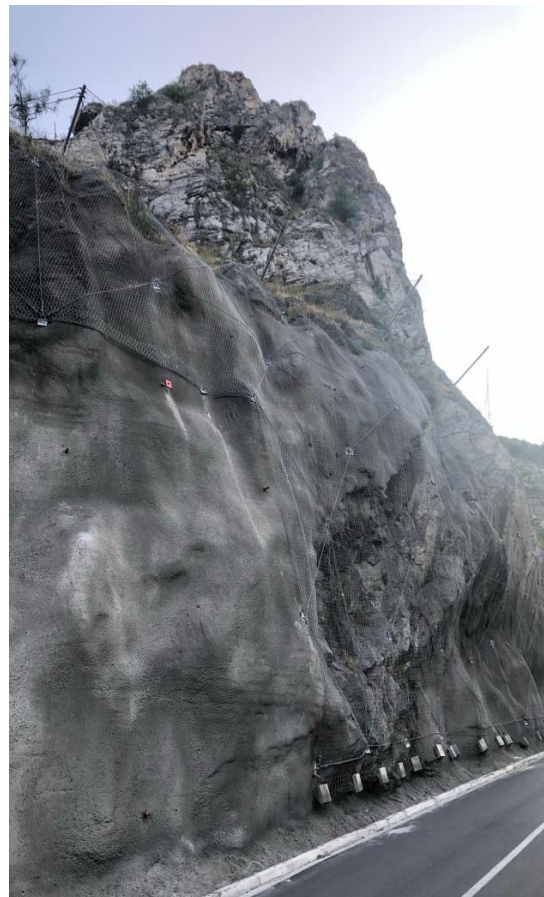
Figure 3. Slope protection, p.c. Cucka, on the regional road R1102 Veles-Gradsko
