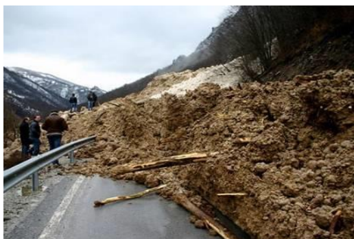
E) Snow and debris avalanche on the road Mavrovo-Debar (2010 year)
