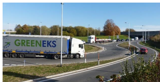
Figure 1. Shear stresses (Fig.1) on the asphalt structure of the roundabout [Hrapović K. 06.11.2015]
