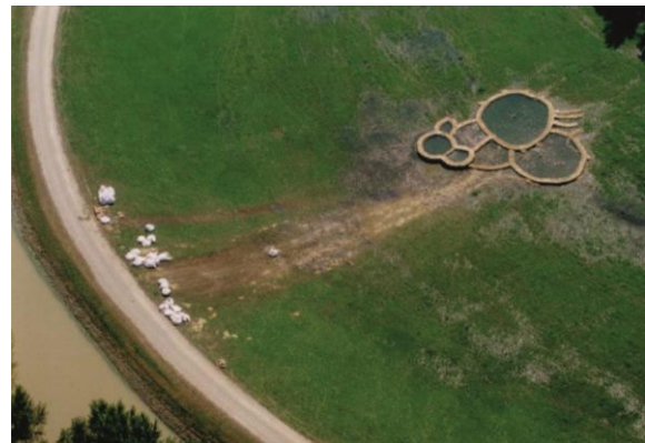
Figure 7. Piping (soil boiling) far away from the dyke and stabilizing measures to reduce the hydraulic gradient (photo: L. Nagy)
