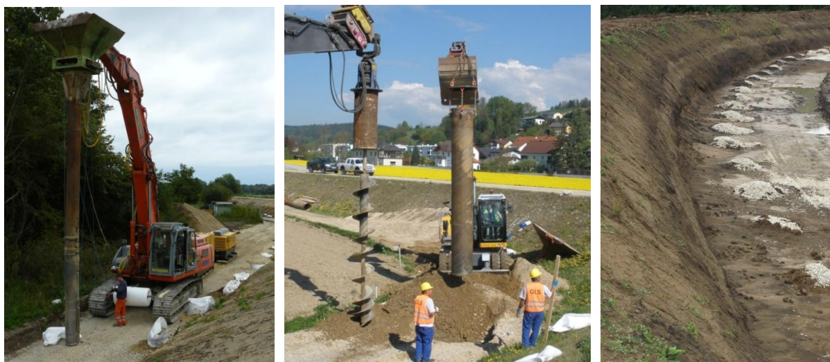
Figure 15. Installation methods of relief drainage columns wrapped in nonwoven geotextile. (left: vibroflotation method; middle: rotary drilling method with casing; right: "infinite" relief column system at the dyke toe)
