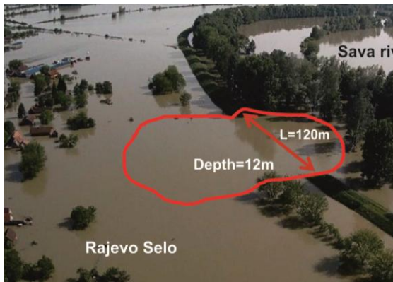
Figure 5. Breach of a Sava River dyke with an extensive scour on the landside (120 x 300 x 12m) due to internal erosion of the ground below the dyke. (Croatian Ministry of Agriculture, 2014)
