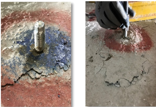
Figure 10. Failure of anchor type 2
