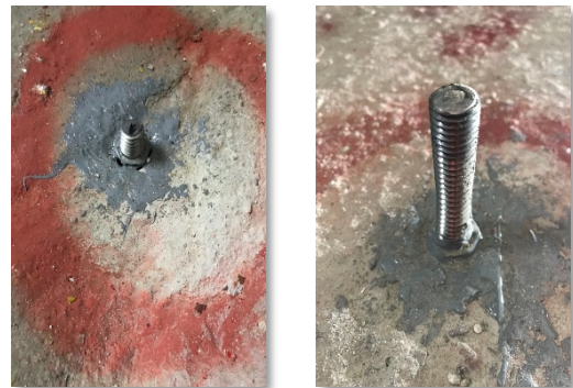
Figure 12. Failure of anchor type 4
