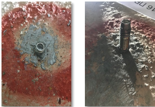
Figure 9. Failure of anchor type 1
