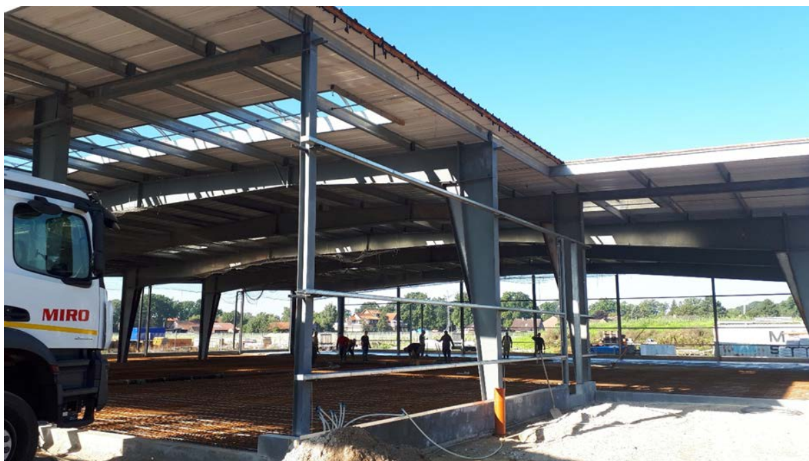
Figure 6. Reinforcement of steel frames
